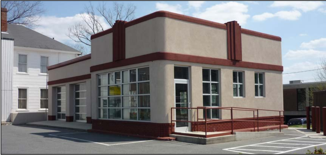
Photo 24: Circa-1935 Gibbon's Esso Station, 623 W. Hillsborough Street (WA-2887). Determined Eligible for NRHP in 1999 and Recently Renovated.
