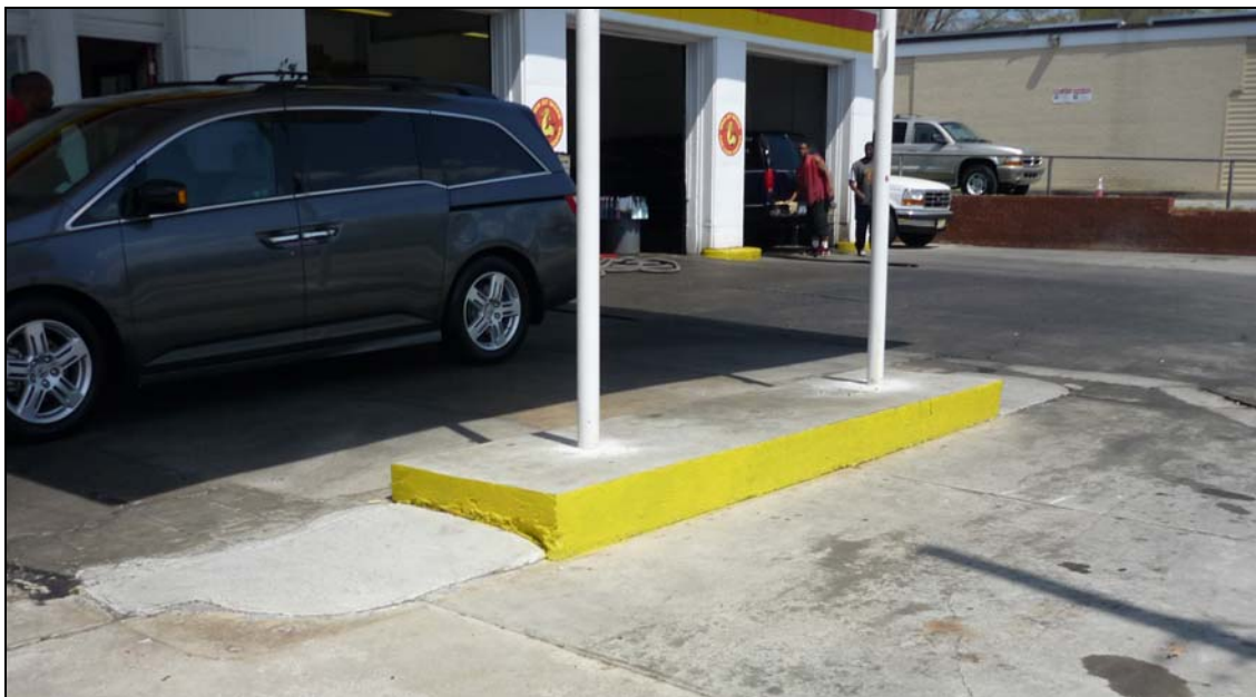
Photo 23: View of Former Pump Island and Canopy Posts, Looking East.
