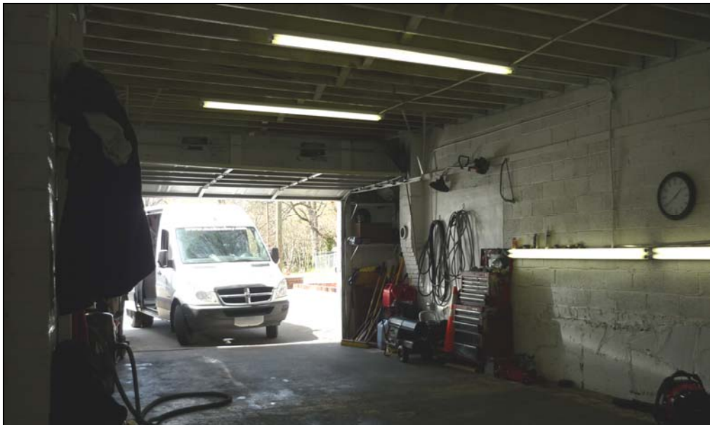
Photo 21: Interior of Rear Addition, View Looking West.
