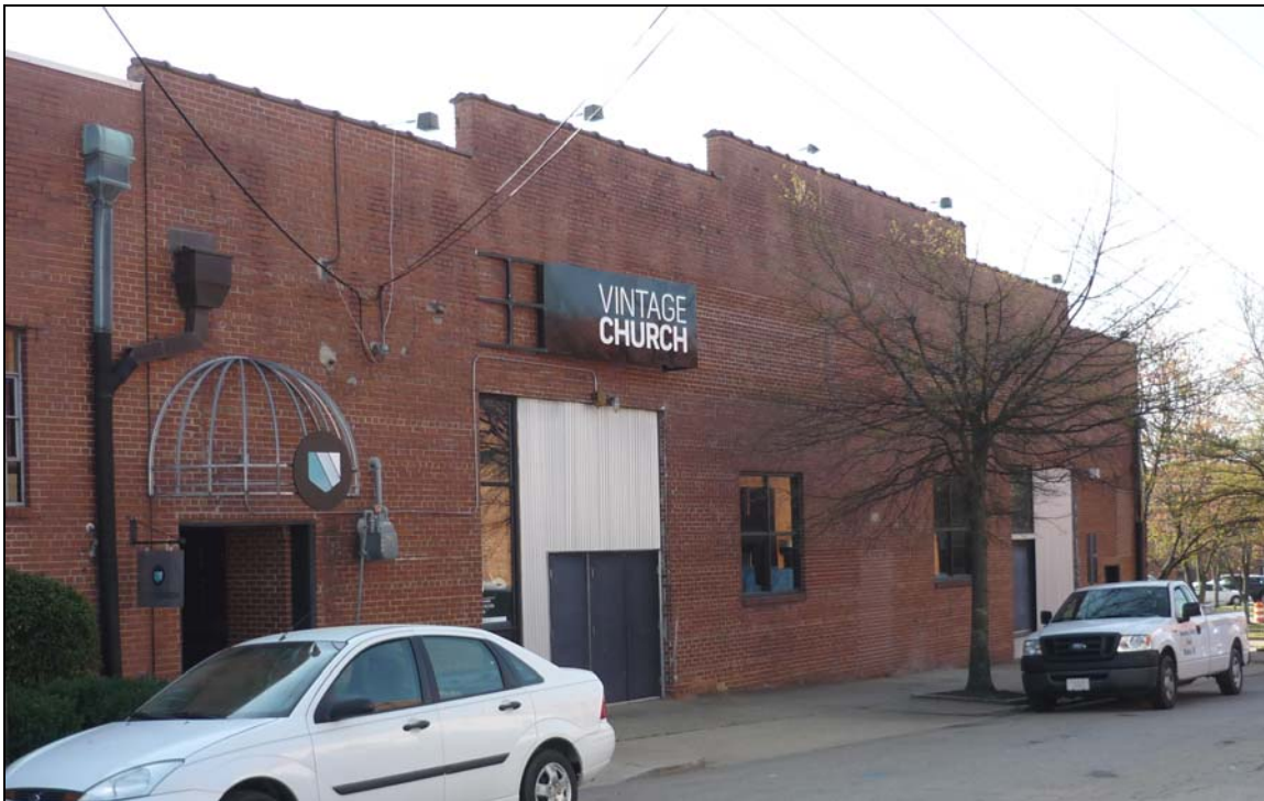
Photo 10: View of West Elevation, 117–121 S. West Street, Looking South Southeast.
