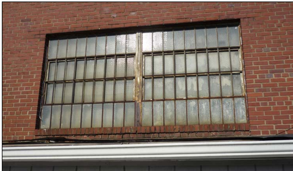
Photo 8: Detail of Original Windows Along East Elevation.
