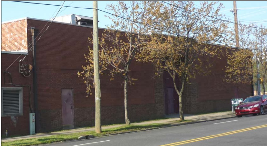
Photo 1: View of North Elevation, 411 W. Morgan Street, Looking Southwest.
