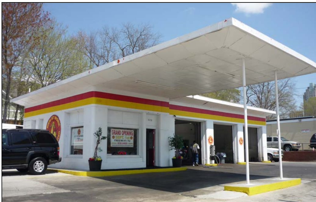
Photo 15: Southwest Oblique, 520 W. South Street.
