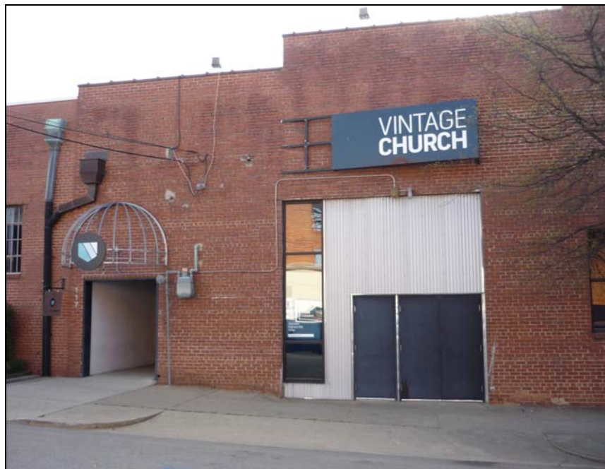
Photo 12: Detail of North Entries to 117 S. West Street, West Elevation. Note curb cuts in sidewalk that facilitated automobile access to the building.
