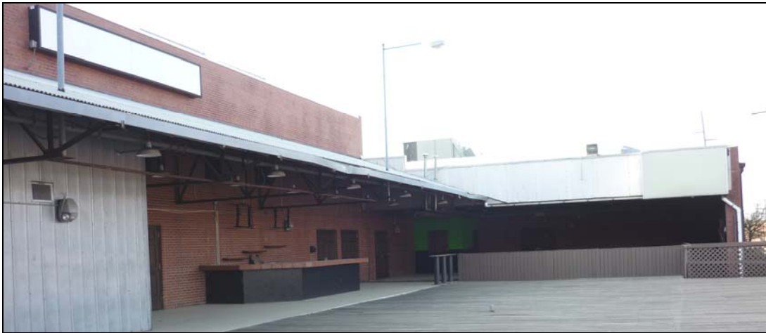
Photo 3: View of Loading Area, West Elevation, Looking South.
