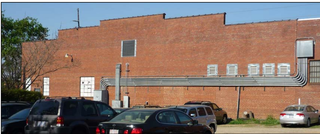
Photo 14: View of Rear, or East, Elevation Looking West-Southwest.
