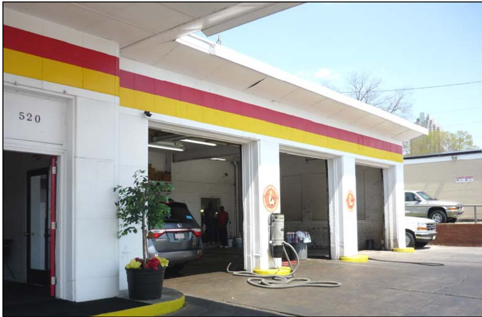
Photo 20: View of Service Area, Looking Northeast.
