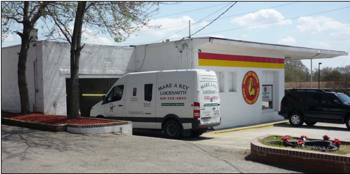
Photo 22: View of Northwest Corner, Showing Garage Entry at Rear Addition.
